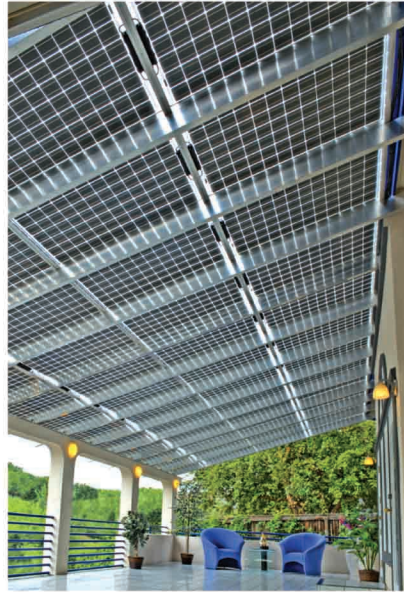
Patio Awning: Solar Living Design Lakewood, CO
